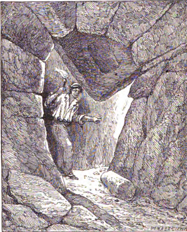
FIG. 107.—Voussoir of Arch fallen through roof of rock-excavated canal. Recovery , p. 105.
